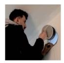
4 Insert the ceramic heat exchanger.
